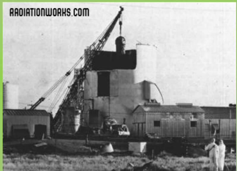
Core removal with crane (radiationworks.com)
