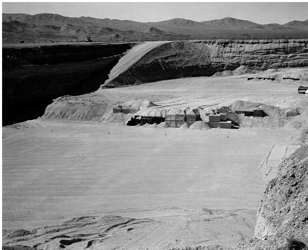
Fig. 35 - Disposal trench at Beatty, NV
