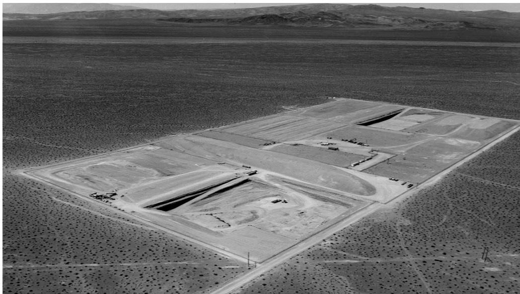
Fig. 34 - Beatty, NV low level disposal facility
