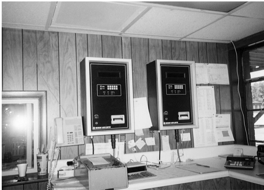
Fig. 47 - Bicon scrap monitor hardware
