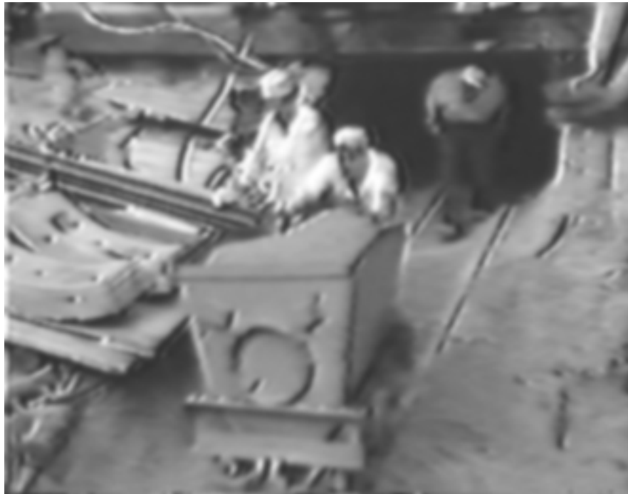
Fig. 36 - Excavating the tunnel beneath the reactor building
