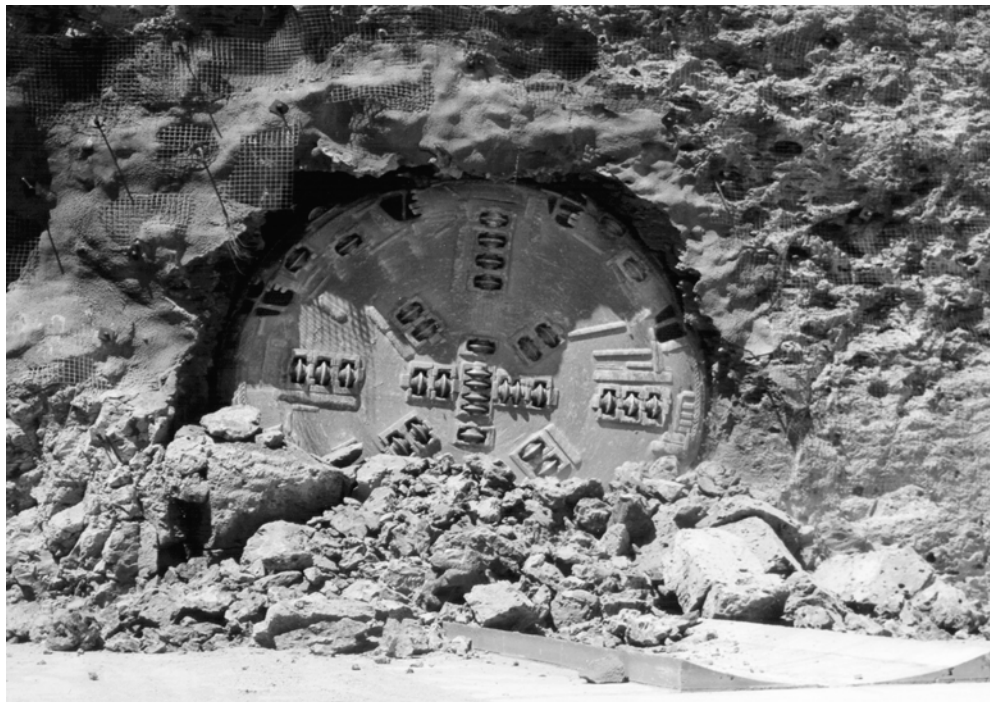
Fig. 54 - The Tunnel Boring Machine emerging from Yucca Mountain
