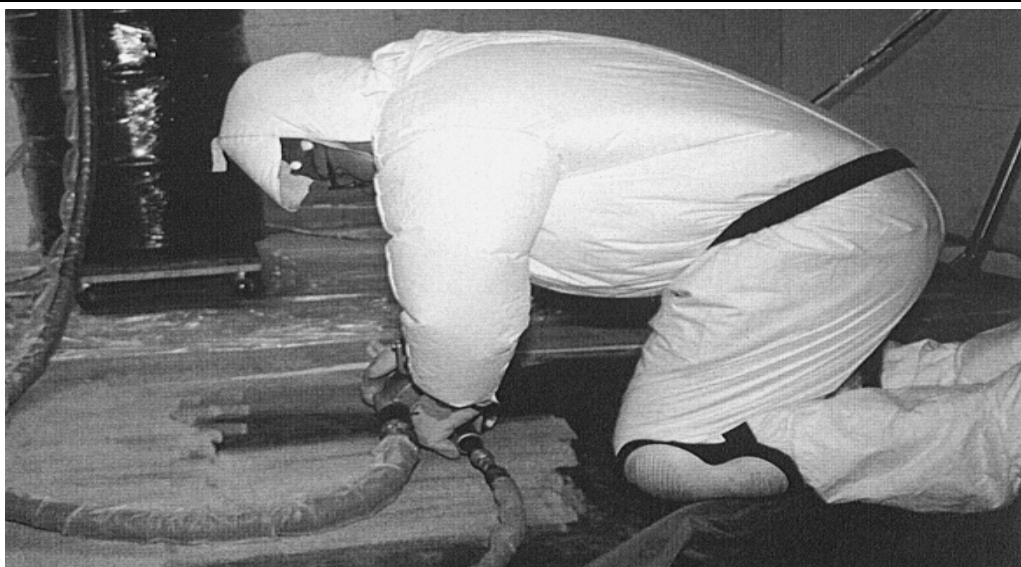
Fig. 38 - A supplied air hood respirator
