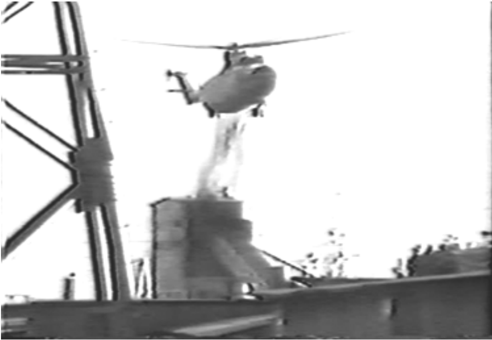
Fig. 33 - Shielding being air-dropped onto the reactor core
