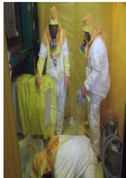
HEPA Filter Removal
