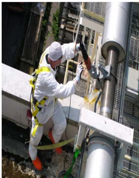
Set Up For Remote Saw Cutting
